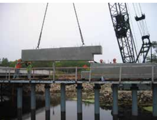
Accelerated bridge construction demonstrated with a precast concrete pier cap.
