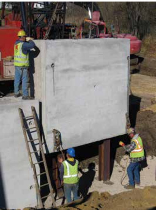
Accelerated bridge construction demonstrated with a precast concrete abutment.
