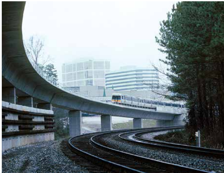
The first precast concrete, segmental, post-tensioned rail transit bridges in the United States were built for the Metropolitan Atlanta Rapid Transit Authority in 1985. Photo: FIGG.
