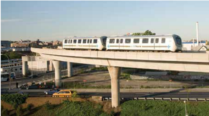
The 8.7-mile-long concrete segmental guideway at JFK International Airport features precast concrete segmental box girders that were erected with four erection trusses working simultaneously using the span-by-span method. Photo: FIGG.
