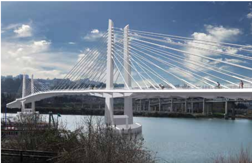
Now under construction, the 1720-ft-long cable-stayed bridge across the Willamette River features three spans of 390, 780, and 390 ft with constant-depth, open-edge segmental girder sections erected using the balanced cantilever method. Rendering: T.Y. Lin International.
