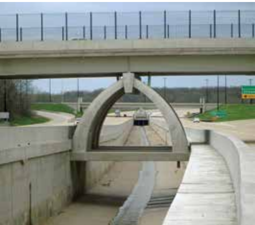
University Bridge on I-74 in Peoria, Ill., features a concrete tied-arch support pier that straddles the Dry Run Creek Flume. The design for the project, which features precast concrete girders, creates an aesthetically pleasing, functional support design.
