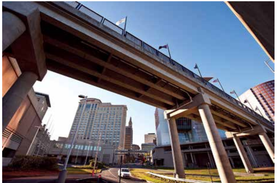
The three-span, 268-ft-long Mayor Mike Peters Pedestrian Bridge in Hartford, Conn., has prestressed bulb-tee girders with a composite precast concrete deck slab. It features two colors of stamped concrete to create a brick-like pattern.
