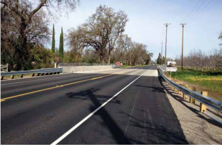
The new 108-ft-long, Craig Creek Bridge, built in 2011 with a crack-free deck and a three-day cure. All Photos: Caltrans.
