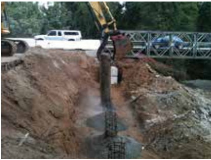
Preplaced cast-in-steel-shell concrete piles were excavated and cut-off to grade.
