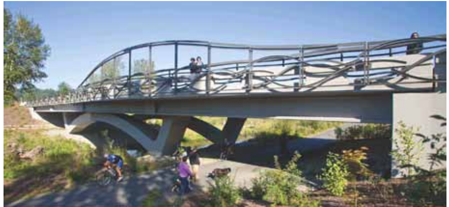
The interweaving decorative railing had to adjust to the vertical and horizontal curves and asymmetrical shape of the bridge, which included sloping bulb-outs on each side to provide lookouts for pedestrians.
