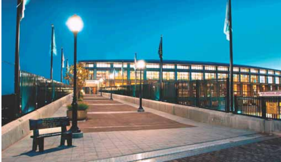
Ornamental lighting, flagpoles, planters, and fields of etched concrete, bordered by bands of integrally colored stamped concrete, were used to enhance the bridge aesthetics because of its prominent location. Photo: Jeffrey Yardis, Corporate Images.
