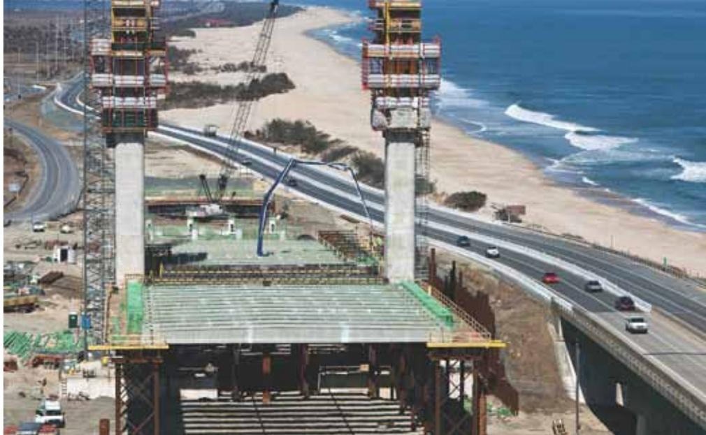
The use of precast concrete floor beams and cast-in-place construction on falsework for the portions of the bridge over land significantly sped construction because work could be completed simultaneously on several different fronts. Photo: AECOM.
