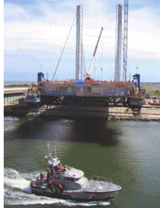
Boat traffic was uninterrupted as cantilever construction of the bridge extended out over the Indian River Inlet. Photo: AECOM.
