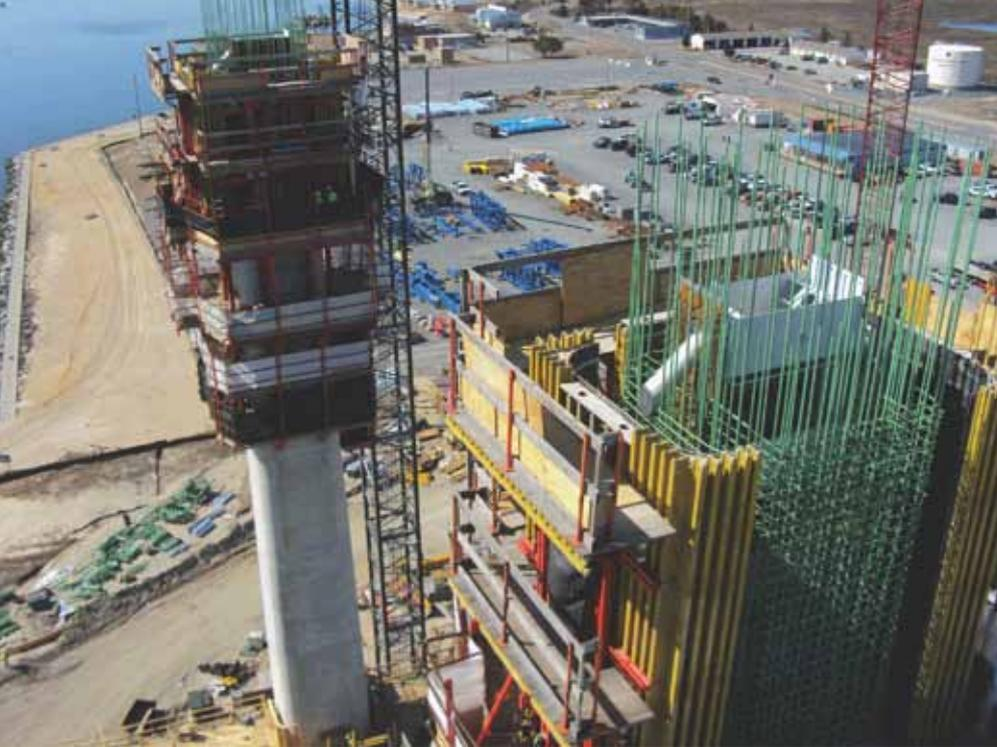
The stays are anchored in the white structural steel anchorage boxes in the pylons. The anchorage boxes take advantage of the high-tensile capacity of structural steel to resist the large horizontal tension resulting from the cable stays, while the vertical compression from the stays is handled by the concrete. Photo: AECOM.
