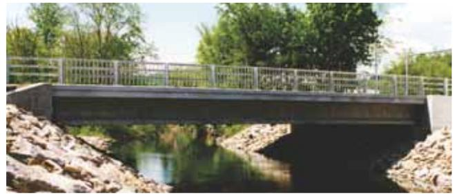
*The Route 104 Bridge, Bristol, N.H., was constructed in 1996. A bridge deck survey 8 years later showed only two longitudinal cracks with a total length of 10 ft. Photo: New Hampshire Department of Transportation.*
