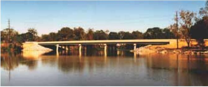
*The Charenton Canal Bridge, La., was constructed in 1999 and inspected 4 years later for cracks in the deck. The only cracks observed were transverse ones in the negative moment region over the intermediate piers. Photo: Louisiana Department of Transportation and Development.*
