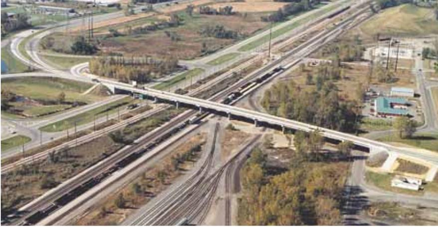
The 10-span bridge on SR 249 over U.S. 12 in Porter County, Ind., features a continuous composite, prestressed concrete bulb-tee design constructed without any joints.
