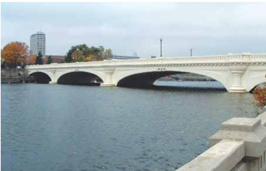
The four-span Jefferson Boulevard Bridge over the St. Joseph River in South Bend, Ind., was rehabilitated by American Structurepoint to retain its original earth-filled concrete Melan-arch design.
