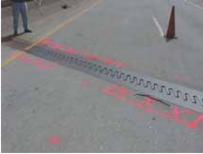
Expansion joint repair before further deterioration occurs.
