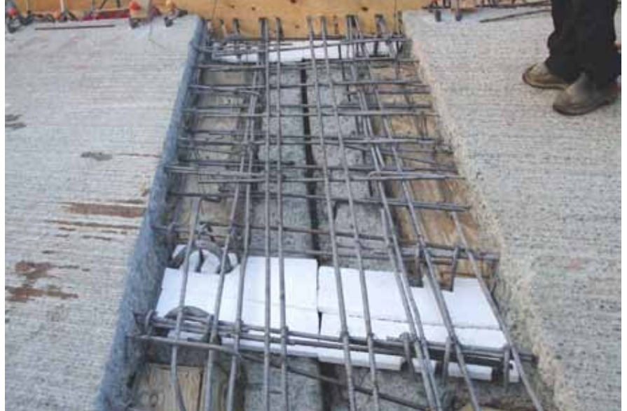
Modular joint replacement in progress.
