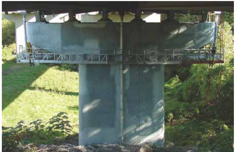
Treatments to restore pier condition.
