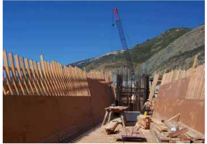
Girder and soffit forms for the first end span are supported on falsework.
