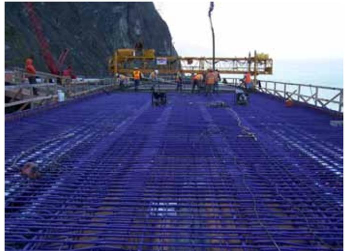
Epoxy-coated reinforcing steel in the deck prior to concrete placement.
