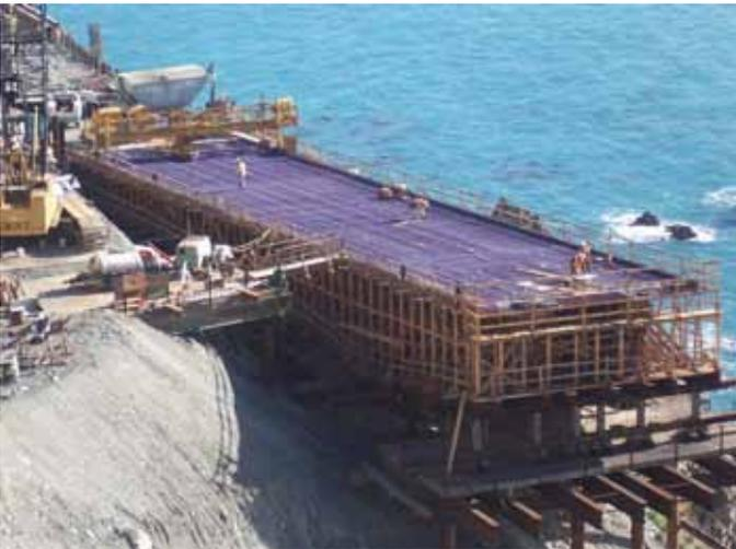
Epoxy-coated reinforcing steel in the deck of the south end span is readied for placement of the concrete. The end spans were formed on falsework.
