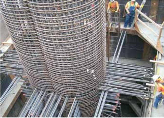
Main bent column reinforcement with partial main bent footing reinforcement being lowered into footing forms.
