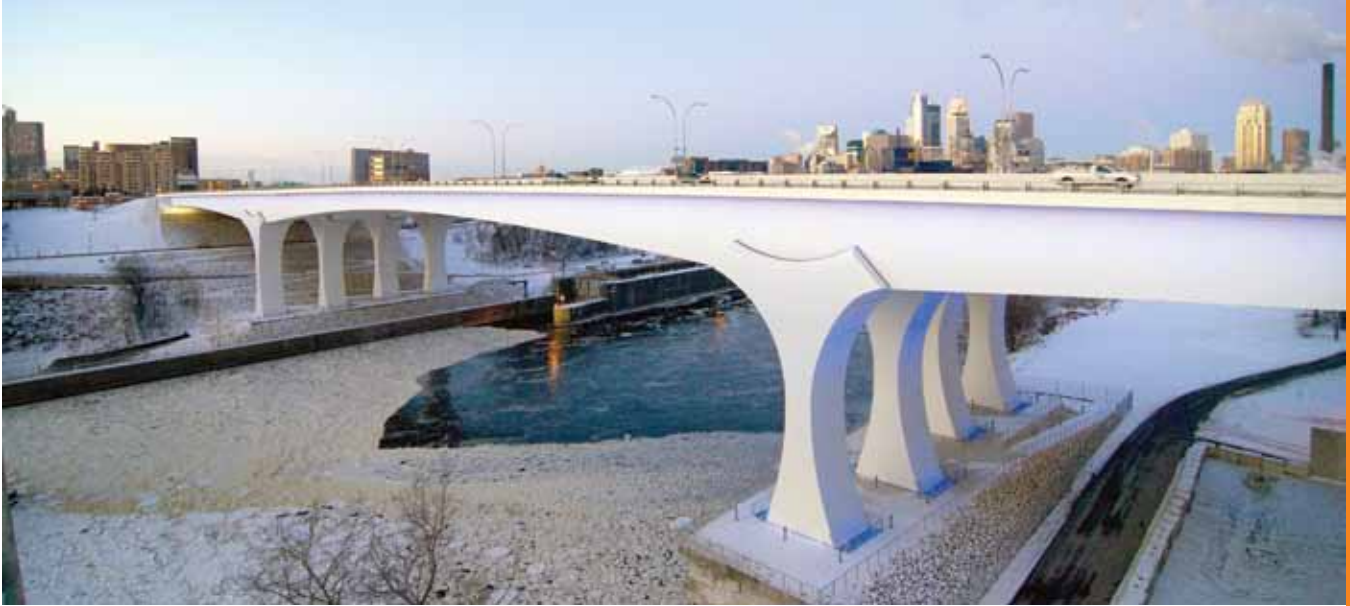
The 120 segments in the main span of the St. Anthony Falls Bridge were erected in 47 days. Photo: ©FIGG.
