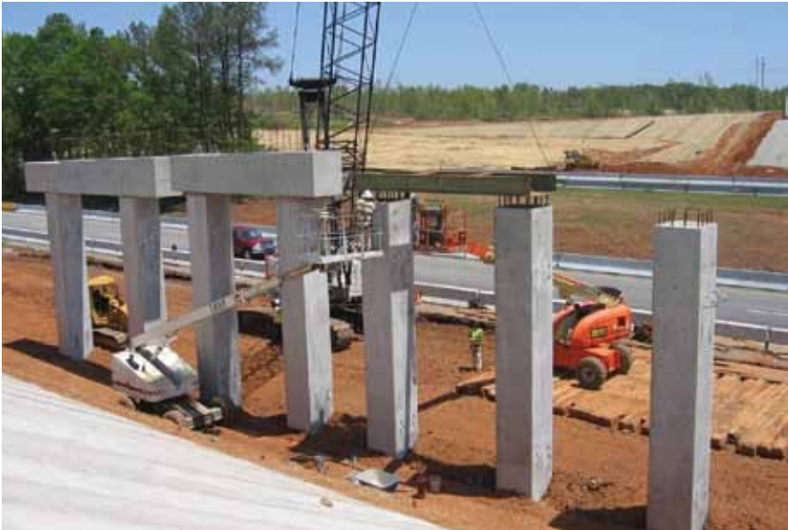
Figure 4. Precast concrete bents were used in Georgia's Highways for Life program.
