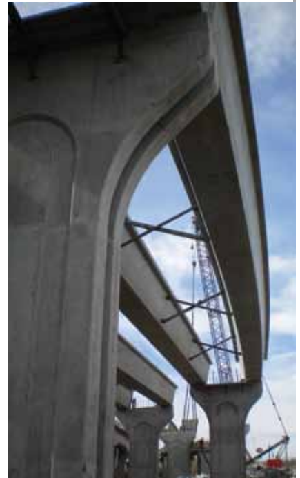
Construction of the IH-25 Viaduct, located in Trinidad, Colo., includes spliced, curved, precast concrete U-girders. Photo: PCI.
