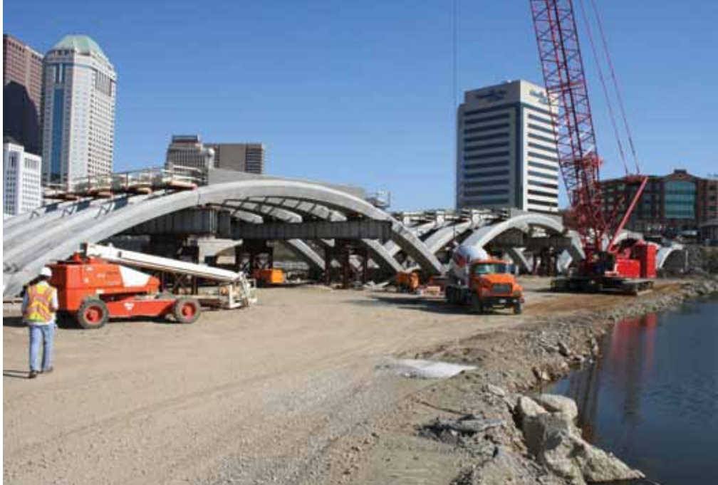
Placing the pier cap closures. Photo: Ohio Department of Transportation District 6.
