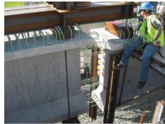
Span segment installation with strongbacks.
