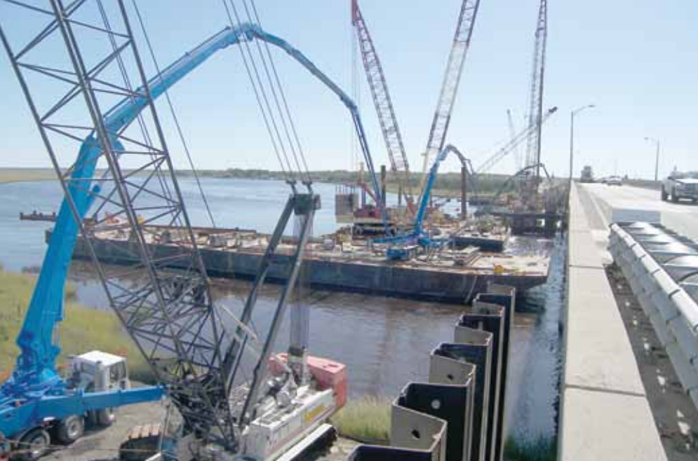
Concrete pumping trucks were used in series to install the self-consolidating concrete in the drilled shafts.
