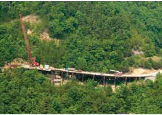
The temporary work trestle construction advances from right to left. A secondary crane provides access for foundations and pier construction.
