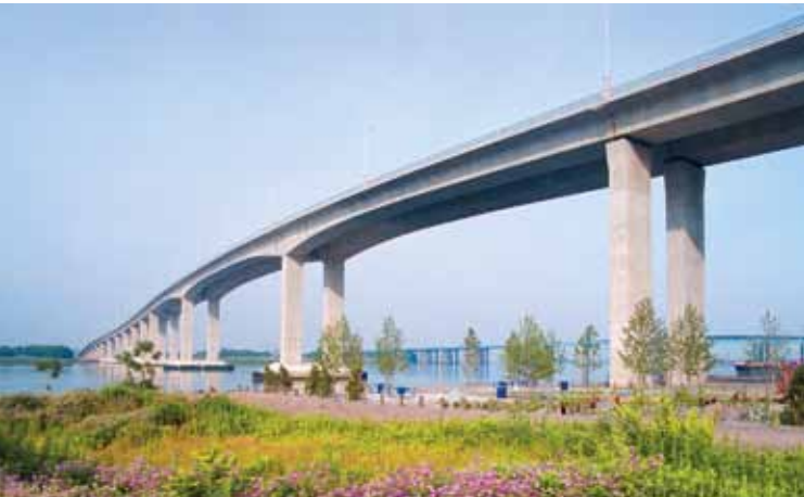
The Victory Bridge in New Jersey was completed more than two months ahead of schedule. Photo: ©FIGG.
