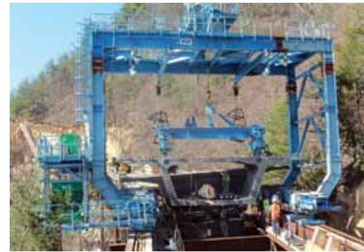
The segment walker places a segment at pier 3.
