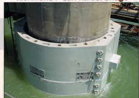
Richmond / San Rafael Bridge
