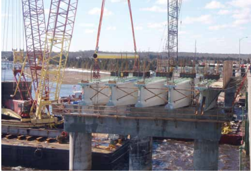
Pier 1 segment installation.
