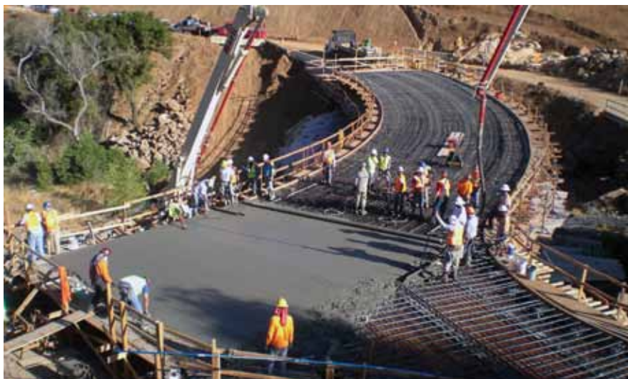
Deck placement using special concrete screed. Photo: County of San Diego.
