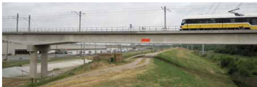
The completed DART Trinity River Bridge over the U.S. Army Corps of Engineers levee.
