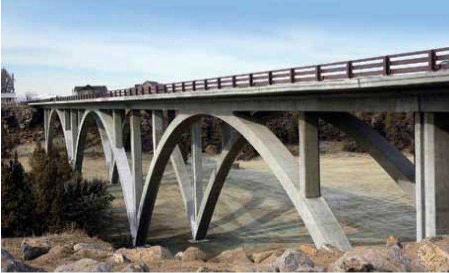
The Maple Avenue Bridge in Redmond, Ore., features cast-in-place concrete arches consisting of two side-by-side ribs fixed at the base while pinned to and continuous across the intermediate footings.
