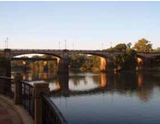
Figure 1. The Dillingham Street Bridge is a Melan Arch, which dates back to 1912. All photos: Georgia Department of Transportation.
