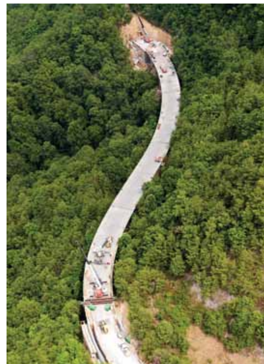
Completed construction of the major bridge elements.
