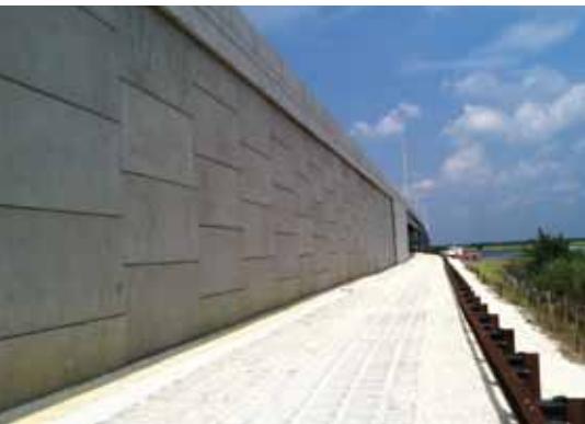
MSE retaining wall and articulated concrete block mattresses were used as an access road.
