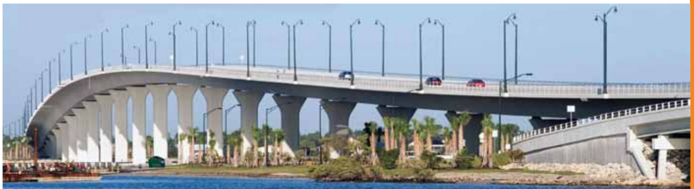
The Earnest F. Lyons Bridge was completed within budget and eight months ahead of schedule. Photo: Jim Schneidermann, PCL.
