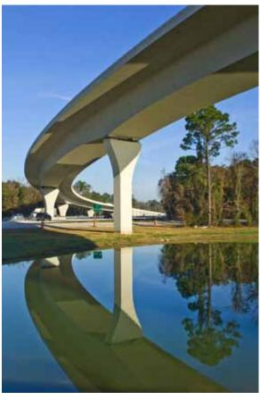
The bridge was completed in September 2010. Variable depth segments were used to increase the span lengths while minimizing materials. Photo: Ray Stanyard Photographer.
