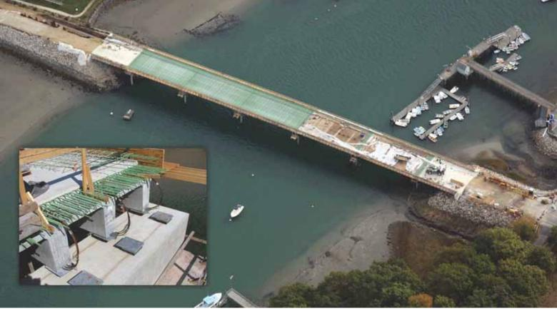
The new Route 103 Bridge over York River in York, Maine, features two 55-ft-long end spans and five 80-ft-long interior spans that use four 36-in.-deep Northeast Extreme Tee (NEXT) beams. The bridge provides the first use of this new girder design, which has wider stems to support higher design loads. Photo: VHB. Inset photo: Dailey Precast.
