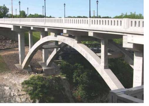
Creative techniques featuring a combination of precast concrete box beams and slabs, plus cast-in-place concrete arches allowed VHB to replicate the look of the original 1913 Lime Kiln Bridge at the Winooski River Gorge in Vermont. The combination replicated the original decorative geometrical features and ornamental railings, while adding safety and durability. Photo: VHB.
