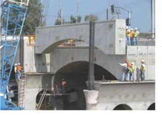
The tops of the piers, which supported the beams, were flared to match the arch shape. Seats on the noses of the piers will receive the precast concrete pilasters. Photo: PBS&J, an Atkins company.
