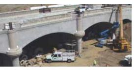
Placement of balustrade railings on beam face projections and architectural precast concrete pilasters on the edges of bents 2, 3, and 4. Photo: City of Rancho Cucamonga.
