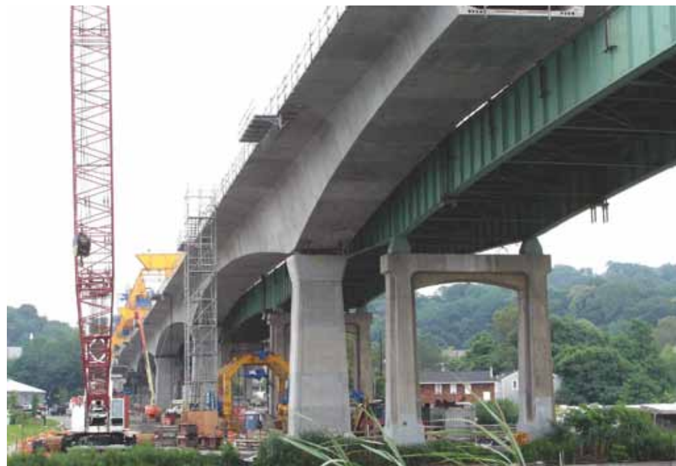
The Roslyn Viaduct used precast concrete segmental construction for both piers and superstructure.
