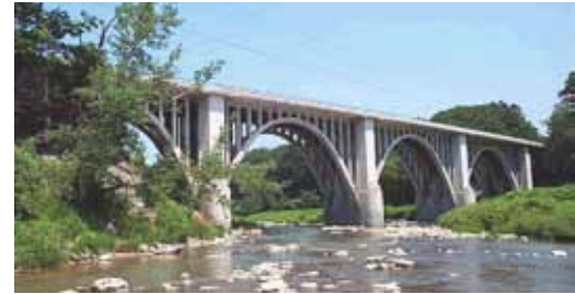
Route 5 over Eighteen Mile Creek in western New York, is an open spandrel cast-in-place, reinforced concrete bridge completed in 1931.
