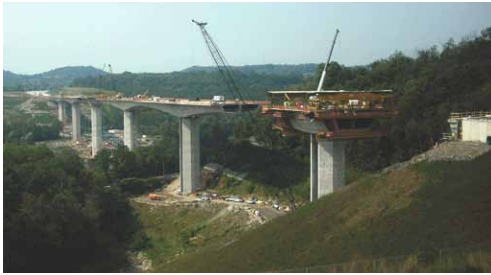
The bridge is constructed using balanced cantilever construction, with seven spans including a main span of 518 ft and piers up to 200 ft tall. Construction of the final cantilevers at Piers 1 and 4 are underway as bridge construction enters the final stages.
