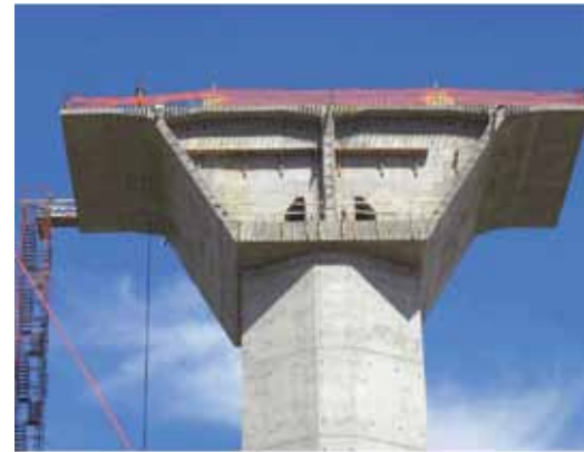
The bridge is constructed using balanced cantilever construction, with seven spans including a main span of 518 ft and piers up to 200 ft tall. Construction of the final cantilevers at Piers 1 and 4 are underway as bridge construction enters the final stages.
