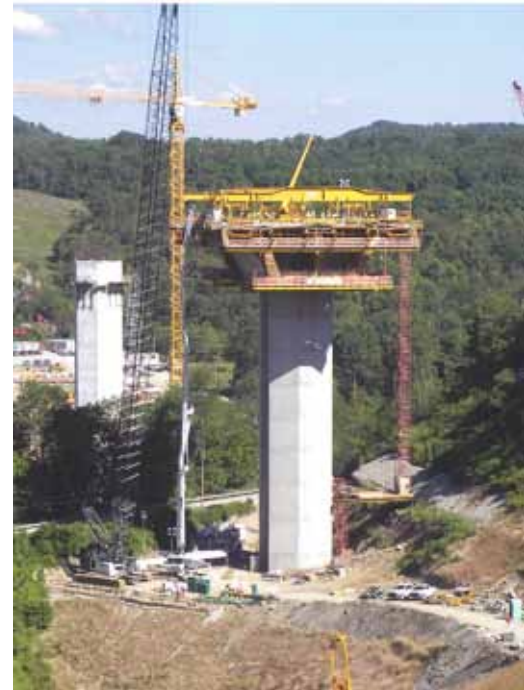
Pier tables begin the balanced cantilever superstructure construction.
