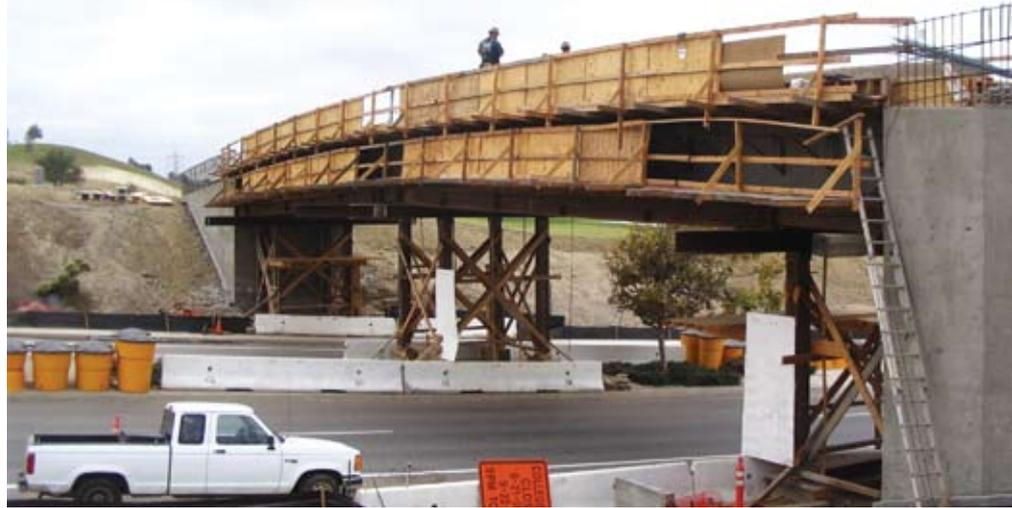
The bridge's deck, curbs, and parapet were all constructed of cast-in-place concrete.
