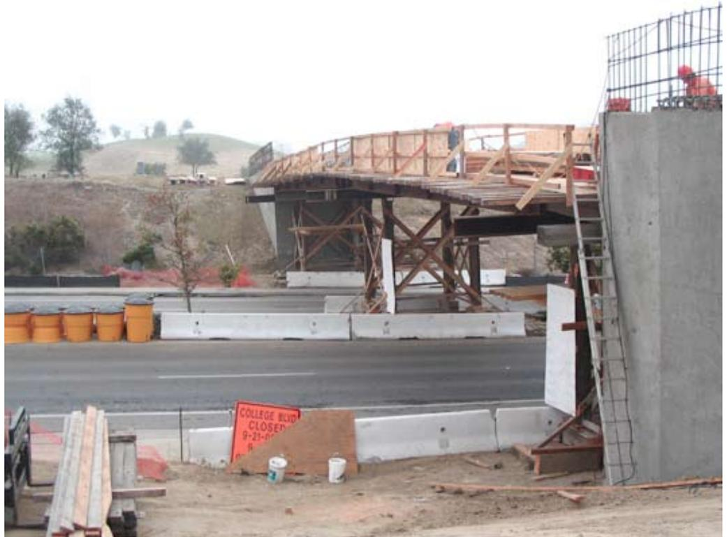
The 123-ft main span and abutments were constructed of 4500-psi, cast-in-place post-tensioned concrete to eliminate the need for a pier in the street's median.
