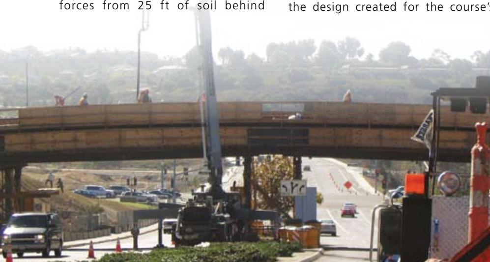
Construction could be handled from the central median on the road below the bridge, avoiding major disruptions to on-going traffic flow.
