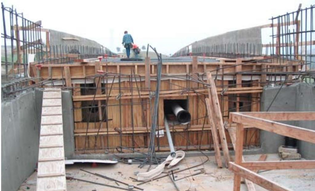
The use of a box girder allows the incorporation of utilities inside the structure, creating a more aesthetically pleasing and protective design.
