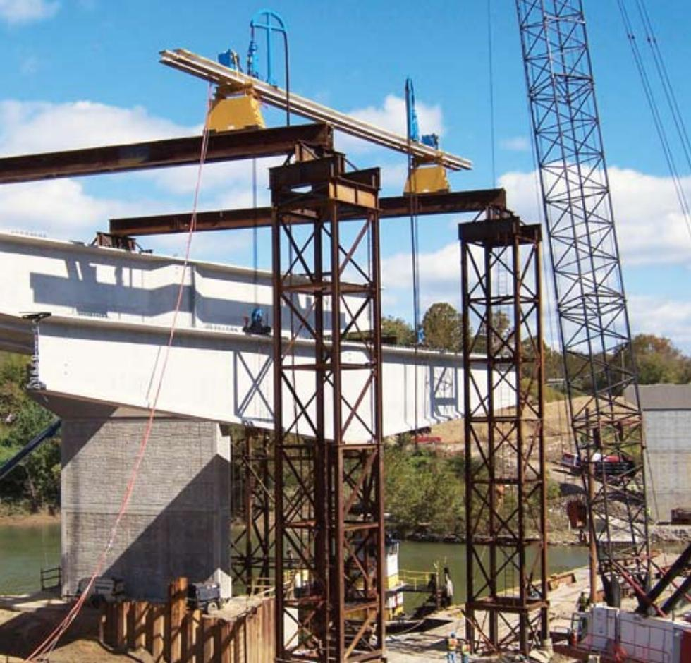
The Kentucky Route 22 project in Gratz, Ky., was redesigned by JSE from a steel-plate girder bridge to a four-span, 909-ft-long spliced bulb-tee girder design that saved about \$800,000 from the previous design. The 325-ft main span provides a record length for construction of this type. Photos: Janssen & Spaans Engineering.
