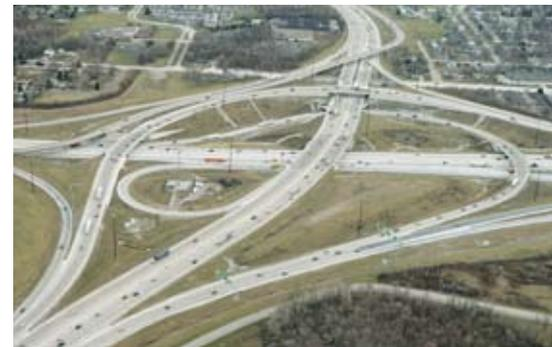
The \$175-million "Super 70" bridge project in Indianapolis involves revamping 6 miles of I-70, comprising all roadway and 23 bridges. In addition, two new bridges were constructed with precast, prestressed concrete I-beams. The design-build project was completed in only 10 months. Photo: © 1800TOPSITE.com.
