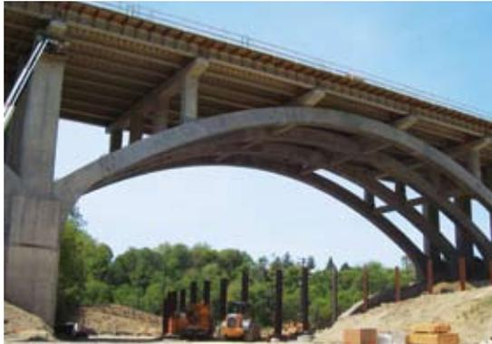
The Fulton Road bridge replacement project in Cleveland, Ohio, features 35 spans of AASHTO Type III precast concrete girders supported on five approach spans and six 210-ft-long precast concrete, post-tensioned arch spans with cast-in-place concrete piers, spandrel columns, and transverse cap beams. The bridge spans a park, the city zoo, a creek, and two active railroad lines.
