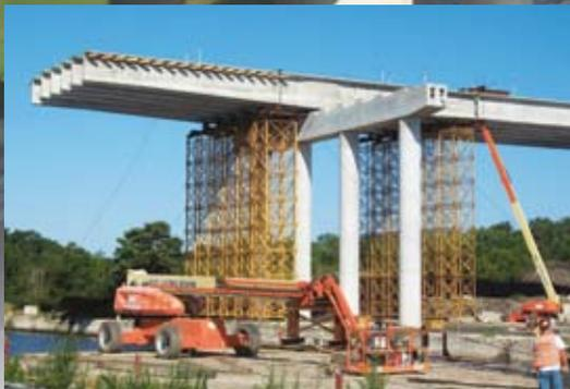
JSE worked under a design-build format to create the design for the Des Plaines River Valley Bridge on I-355 in Lemont, Ill. The bridge features a combination of 18 spans with simple pretensioned concrete beams and 17 spans with post-tensioned spliced girders over its 1.3-mile length. Photos: Illinois State Toll Highway Authority.
