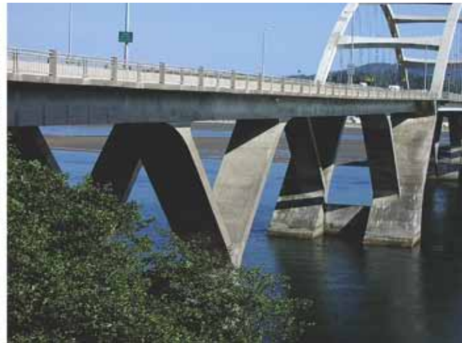
The 1936 Alesha Bay Bridge, shown on left, at Waldport was one of five bridges built simultaneously under a large Public Works Administration project that eliminated five ferries along the Oregon Coast Highway. Designed by Conde B. McCullough and his staff to complement their natural settings, all five bridges included reinforced concrete arches. The Alesha Bay Bridge was replaced in 1991 with a new bridge, shown on right, that features post-tensioned concrete box-girder approaches. Photos: Oregon Department of Transportation.
