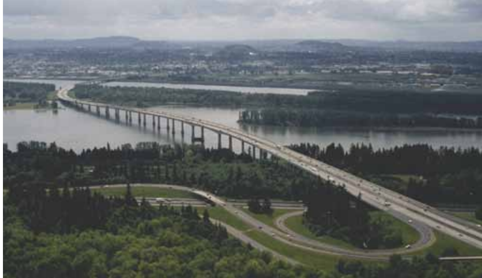
Seen from the north, the 1982 Glenn L. Jackson Memorial Bridge across the Columbia River at Portland was touted as the "first of a new generation of large segmental bridges." Photo: Oregon Department of Transportation.
