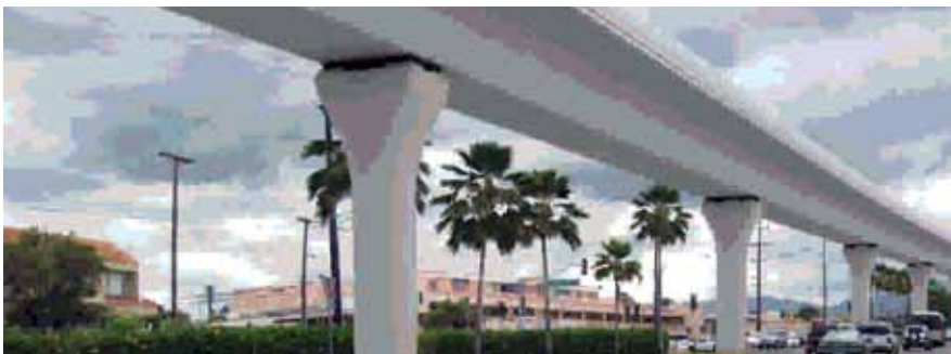
The City and County of Honolulu placed an emphasis on sustainable solutions for Honolulu's new 20-mile elevated rail line. Concrete offered many advantages to meet the needs of the project. Preliminary rendering: Kiewit, HNTB, and FIGG.
