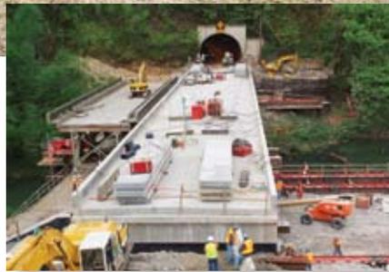
In their quest to maintain mobility, the Oregon DOT designed Elk Creek Crossing No. 4 on OR 38 to be constructed alongside the existing bridge. In one weekend traffic closure, the old bridge was slid aside and the new concrete bridge moved into place with the use of self-propelled modular transporters. Photos: Slayden Construction Group Inc.
