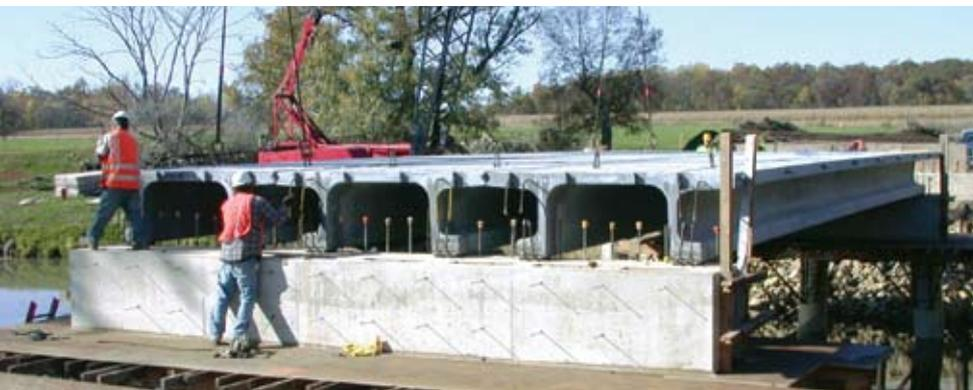
The optimized "Pi" beam developed for the Federal Highway Administration and first used in Buchanan County, Iowa, has a concrete design strength of 21,500 psi. The full structural depth of the deck is just 4<sup>1</sup>/<sub>8</sub> in. Photo: Iowa DOT.
