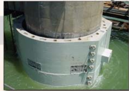
Richmond / San Rafael Bridge
