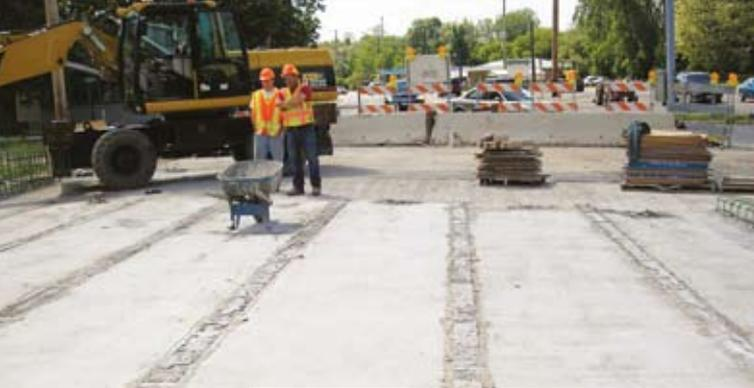
The joints were overfilled to account for some settling in the UHPC mix. The excess was ground off later.
