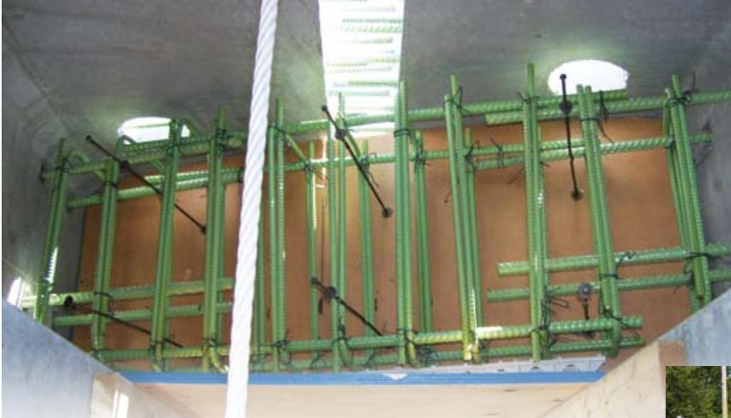
The 6-in. wide joints were created by extending epoxy-coated reinforcing bars 4 in. or 6 in. from the edge of each flange, offset longitudinally so they would not meet each other, and filling the joints with ultra-high-performance concrete.
