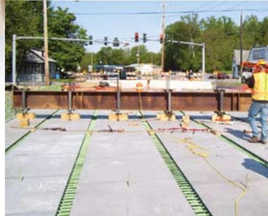
After the beams were set, a jacking system was used to even out the camber between the beams, so they were as level as possible for the waterproofing membrane and overlay.
