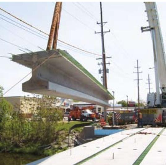
The bridge consists of eight precast concrete deck bulb-tee girders that were erected to close tolerances despite a variety of logistical needs.
