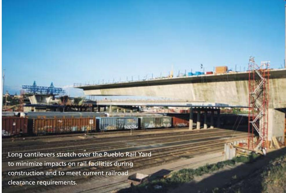
Long cantilevers stretch over the Pueblo Rail Yard to minimize impacts on rail facilities during construction and to meet current railroad clearance requirements.
