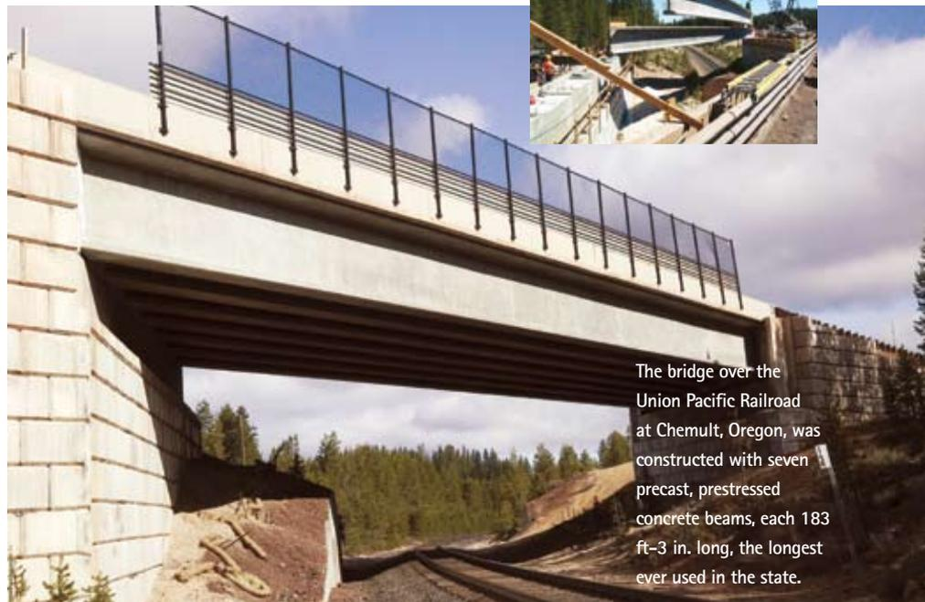
The bridge over the Union Pacific Railroad at Chemult, Oregon, was constructed with seven precast, prestressed concrete beams, each 183 ft-3 in. long, the longest ever used in the state.
