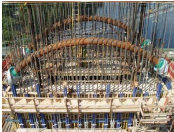
Two of the cradles positioned within the pylon are shown prior to casting. The 20 cradles in each of the pylons carry the strands (from 41 to 73 per stay) through the pylon, eliminating the need for anchorages within the pylon.
