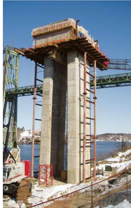
Lower pylon structures were cast in 15-ft lifts. Construction-lift articulations replicate an impression of large granite blocks to complement the actual granite at the entrance to the pylon observatory.
