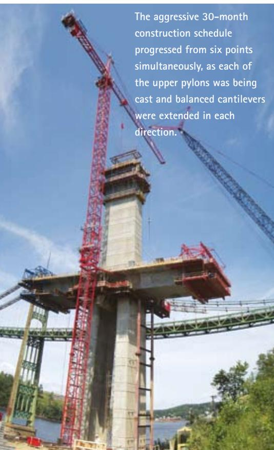
The aggressive 30-month construction schedule progressed from six points simultaneously, as each of the upper pylons was being cast and balanced cantilevers were extended in each direction.
