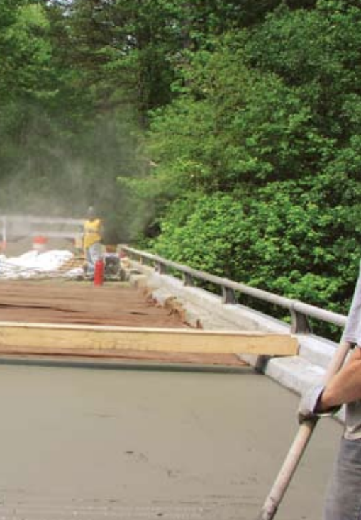
At least 7 days of curing with wet burlap and plastic sheeting are essential for bridge decks.
