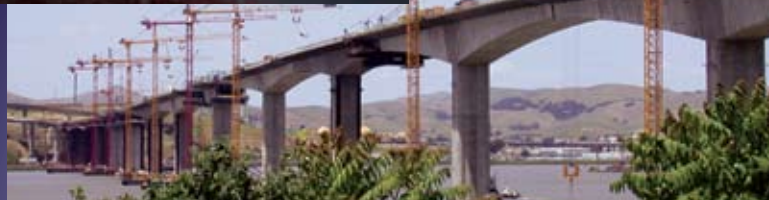
Benicia-Martinez Bridge—California Lightweight concrete box girder superstructure.
