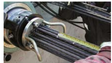
After the concrete has gained strength, the cables are post-tensioned and strand elongation measured.
