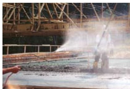
Fog misting can be used to reduce the evaporation rate.
