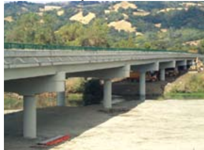
Russian River Bridge, Sonoma County (Precast, prestressed and post-tensioned double-tee superstructure used as an emergency replacement).
