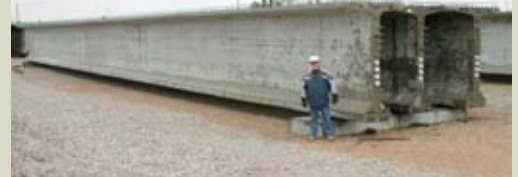
Precast, prestressed concrete, 190-ft-long I girders with WWR shear reinforcement.
