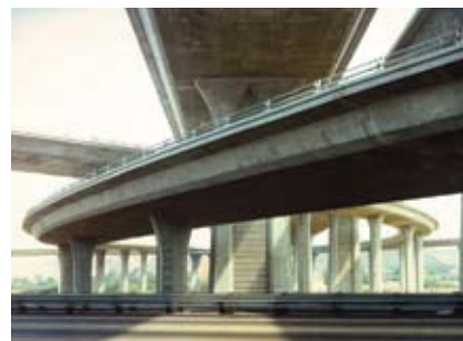
Mission Valley Interchange, San Diego County (Multi-span box girders on single column bents).
