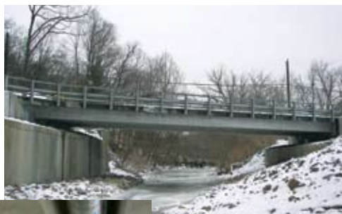
Spread box beams provide an economical solution for the new Zion Hill Bridge.
