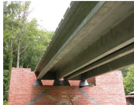
Ultra-high performance concrete, as used in this test bridge for FHWA, is a new material for bridge construction. Photo courtesy of Ben Graybeal, FHWA.
